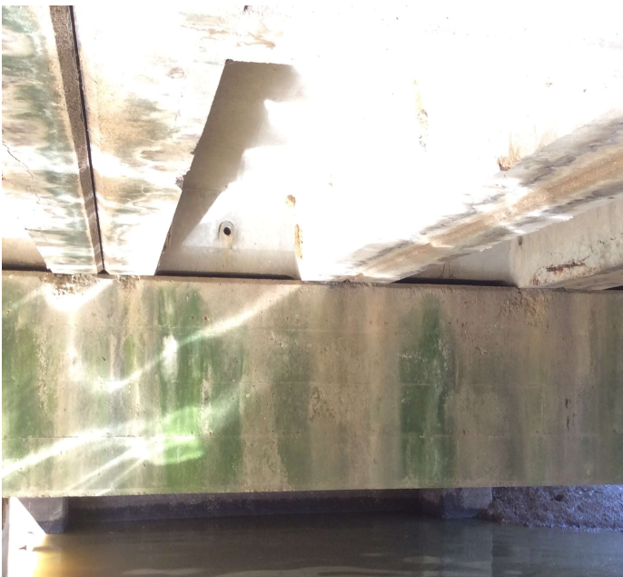
PHOTO 1 Description Shallow spalls in the bearing areas under the stems of channels. Bent 2 in Span 2 pictured.
