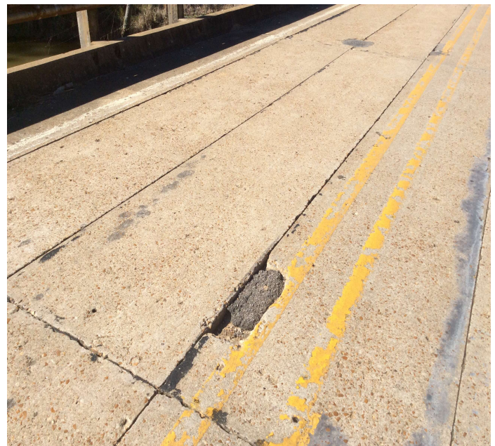
PHOTO 2 Description Pre-cast concrete channels have spalls on the driving surface of the deck. Span 3, Unit 4 at Bent 4 pictured.
