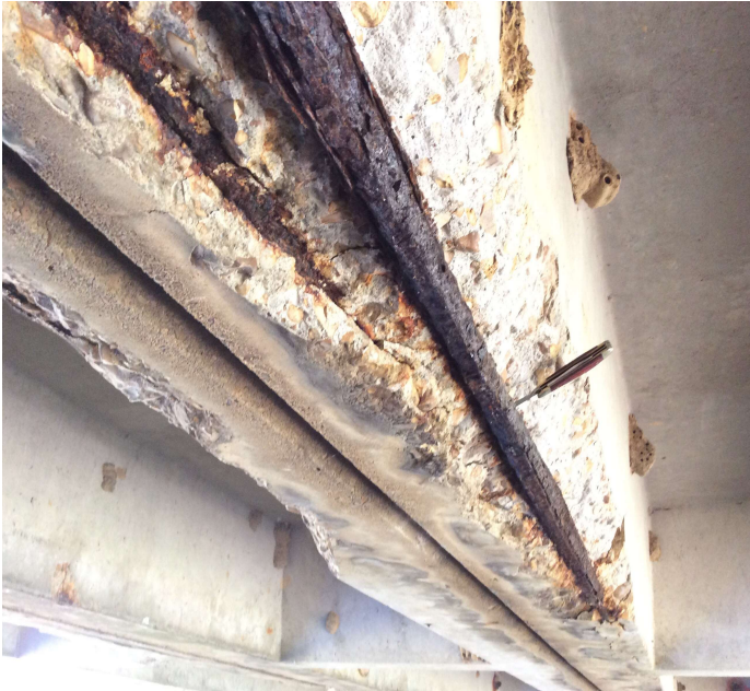
PHOTO 5 Description Span 3, Unit 4 has exposed reinforcing steel that has caulking smeared over the reinforcing steel as a type of repair. The exposed primary longitudinal reinforcing steel in the stem of Span 3, Channel 4 measured 1/16" at this inspection and lost its bond with the concrete along a 5' long area.
