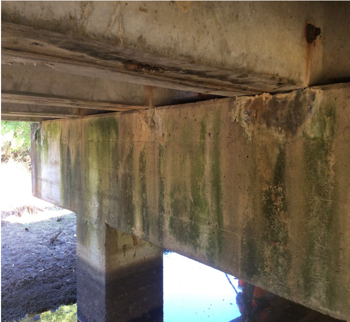
PHOTO 3 Description Shallow spalls in the bearing areas under the stems of channels. Some spalls have been covered with caulking by maintenance forces as a type of repair. Bent 4 in Span 3 pictured.
