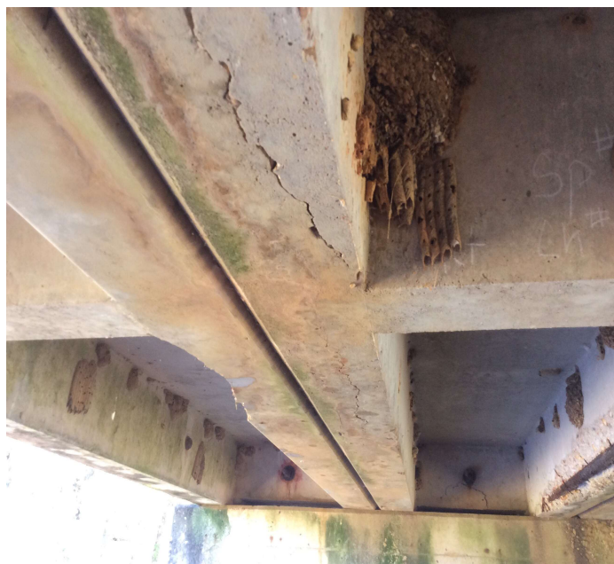
PHOTO 1 Description Numerous areas with longitudinal cracking visible on the bottom surface of the channel Unit legs.
