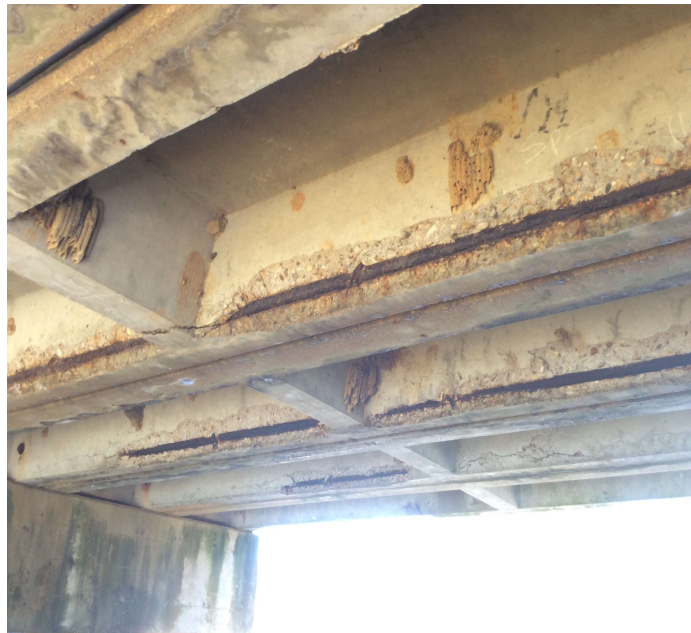
PHOTO 3 Description Numerous areas with longitudinal concrete cracking, spalling with exposed reinforcing steel & delamination in the stems of Channels. -Span 2-Lt Leg of Channel 2 -Span 2-Lt Leg of Channel 3 -Span 2-Lt Leg of Channel 4
