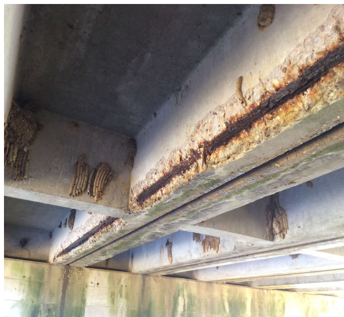
PHOTO 2 Description Numerous areas with longitudinal concrete cracking, spalling with exposed reinforcing steel & delamination in the stems of Channels. -Span 1-Rt Leg of Channel 2 pictured.
