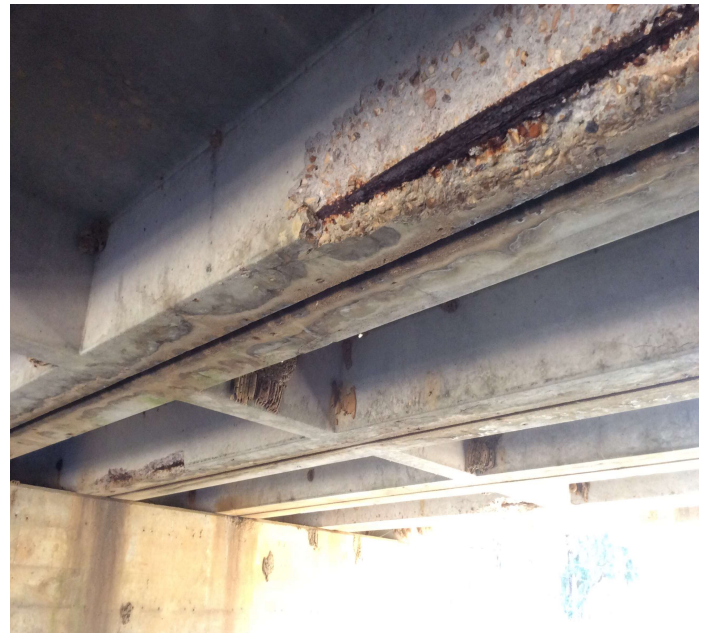
PHOTO 4 Description Numerous areas with longitudinal concrete cracking, spalling with exposed reinforcing steel & delamination in the stems of Channels. -Span 4-Rt Leg of Channel 3 -Span 4-Rt Leg of Channel 4 -Span 4-Rt Leg of Channel 6
