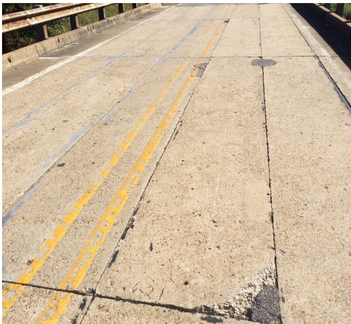
PHOTO 1 Description Pre-cast concrete channels have spalls on the driving surface of the deck. Span 2 Units 4 & 5 pictured.
