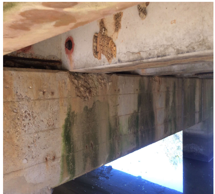
PHOTO 2 Description Shallow spalls in the bearing areas under the stems of channels. Bent 3 in Span 3 pictured.
