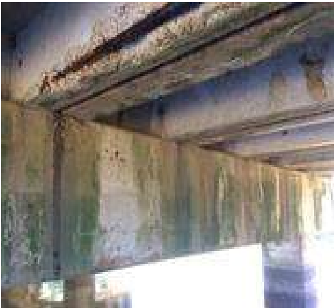
PHOTO 4 Description Shallow spalls in the bearing areas under the stems of channels. Bent 2 in Span 1 pictured.
